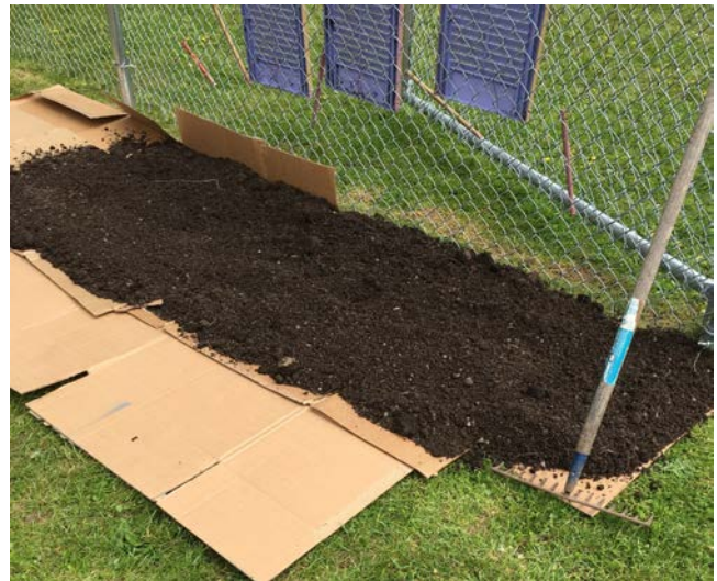
Sheet mulching in progress utilizing cardboard and mulch to smother grass and establish a new garden, RCSD School #29
