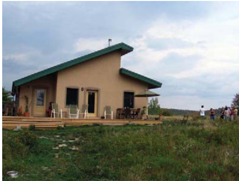
Participants on the 2007 Green Buildings Open House examine the energy-saving features of the Newfield home of Pat Floyd and Kate Halliday. Over 600 people visited the 26 homes and businesses that were part of this year’s tour.
